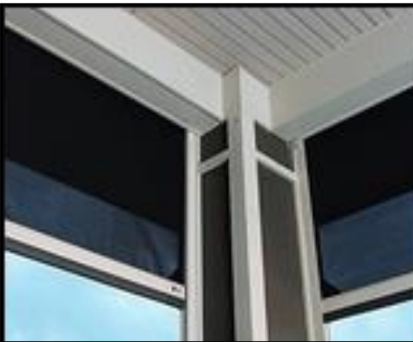
Wood Clad Column
